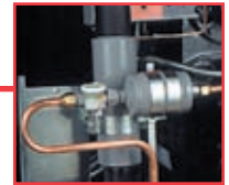
LIQUID LINE FILTER/DRIER
