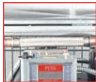
LIQUID LINE VIBRATION ABSORBER (SEMI-HERMETIC ONLY)
