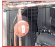
HEAD PRESSURE CONTROL (FLOODING VALVE)
