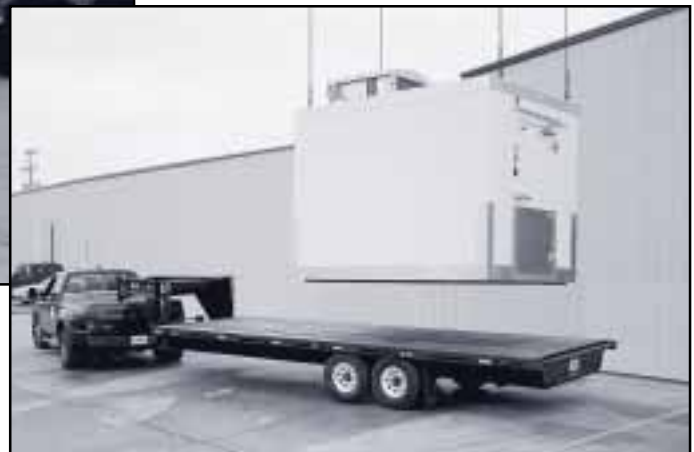
(Above) Each Ready-Bilt is delivered on a gooseneck truck. (Right) Ready-Bilt walk-ins are set in place using a crane, boom-lift or forklift depending on the job situation.
